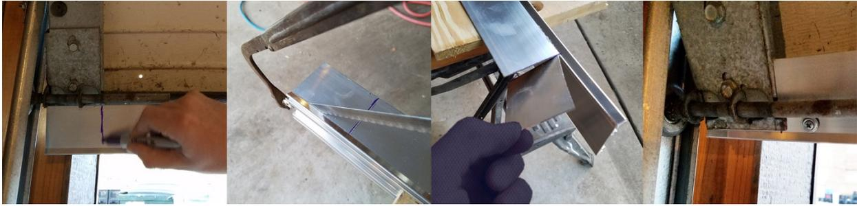
5A. Apply WD-40, silicone spray, or dish soap, into the brush & T-Rubber channels.
