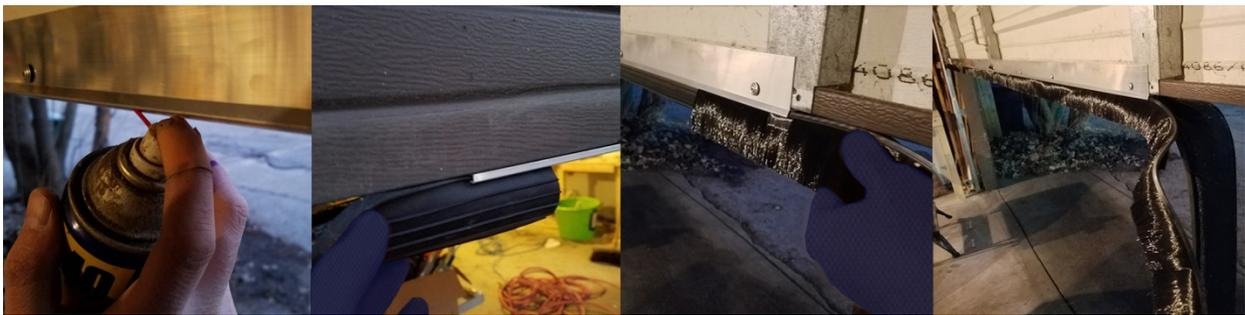
7. Take the loose retainer and cut to fit remaining space. Lubricate channels, as before. Carefully, feed the T-Rubber and Brush Seal into the retainer, pulling the retainer & seals "together", until "loose" retainer sits flush against mounted retainer:
